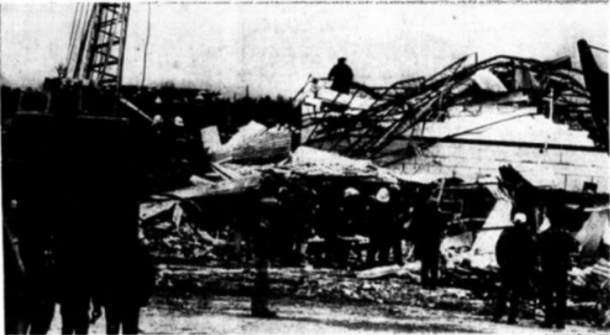
Rescue workers survey the remains of a store in the Northwood Shopping Center in Bennettsville, S.C.
