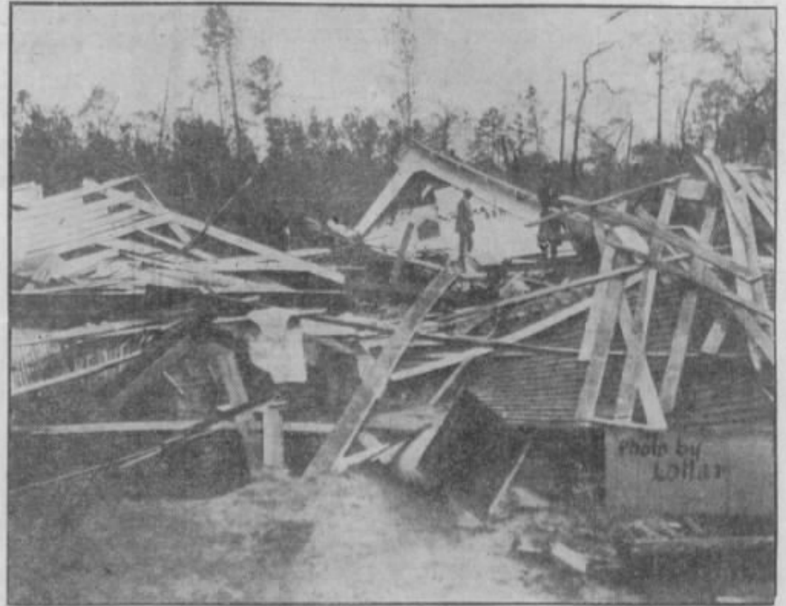
The wrecked Horrell Hill school house, in lower Richland, where four children were killed and many injured by the tornado yesterday.
