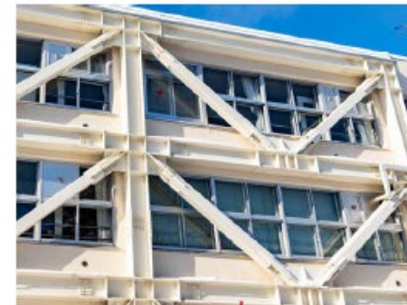
Retrofitting a building by adding a steel brace frame to a structure's exterior helps prevent movement and building collapse during an earthquake.
