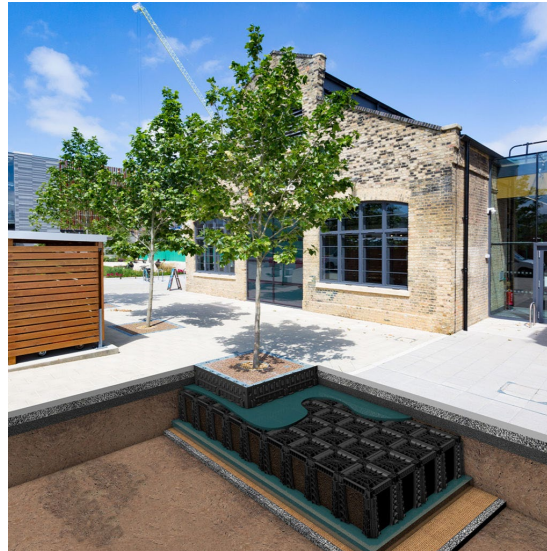
Stormwater Trees & Tree Trenches
