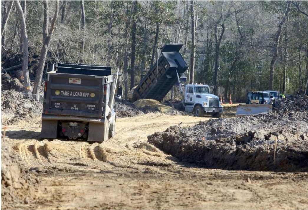
Contractors clear land and build roads for a new subdivision on Johns Island's River Road. Brad Nettles/Staff
